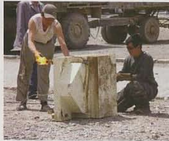
Welding up petrol tank Mongolian-style
